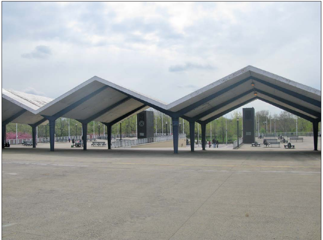
Passerelle Ramp, view south to Flushing Meadows Corona Park 12
