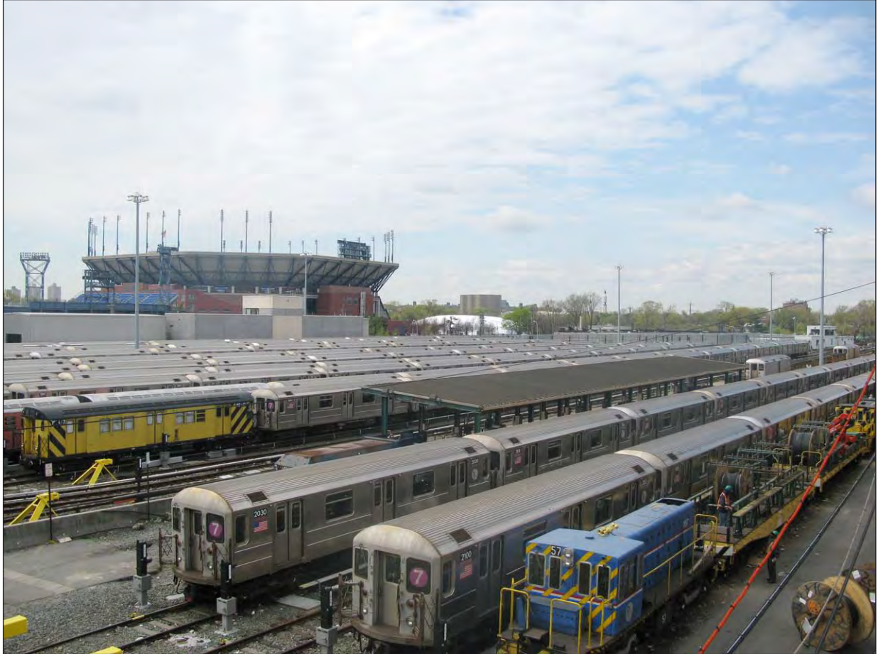
View from Passerelle Ramp to project site 25
