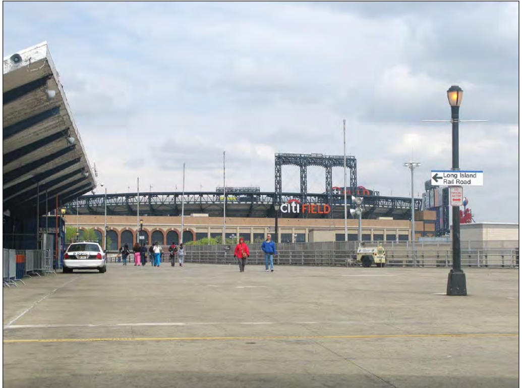
Passerelle Ramp, view north to Citi Field 11
