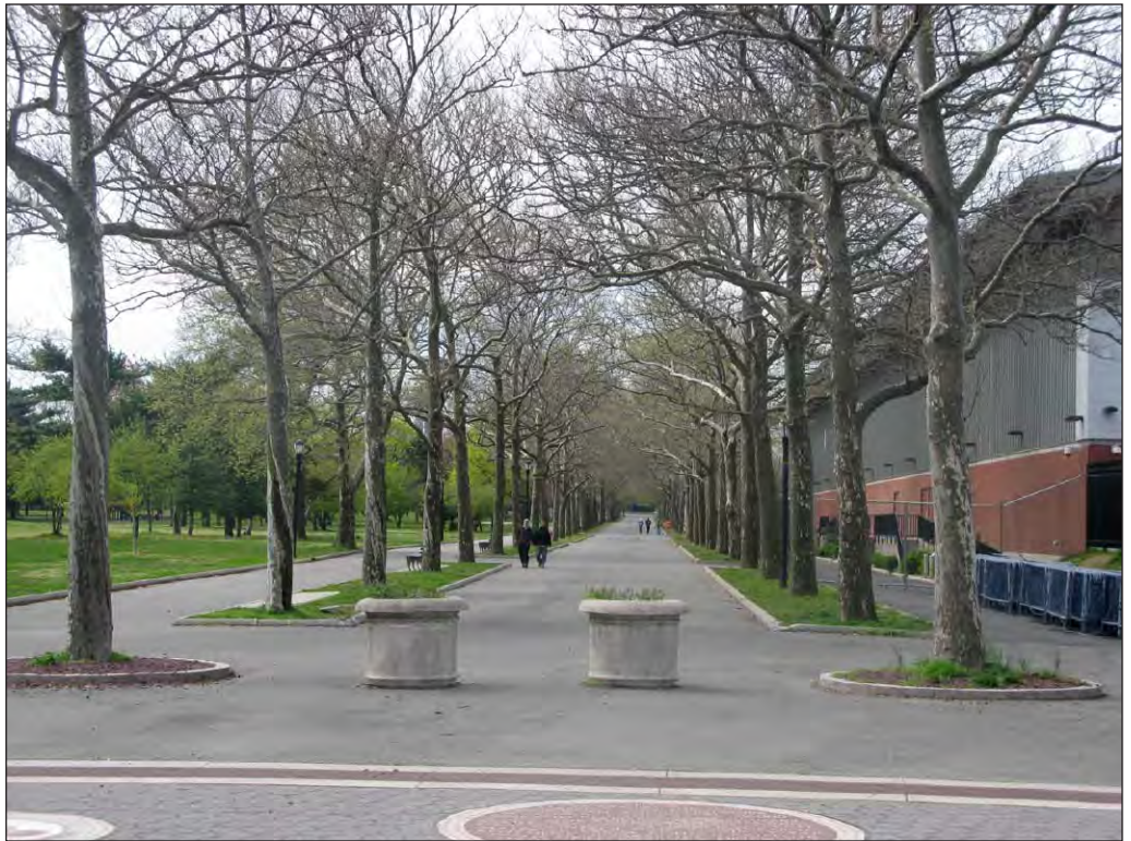
Indoor Tennis Center, view southwest along Path of the Americas 4
